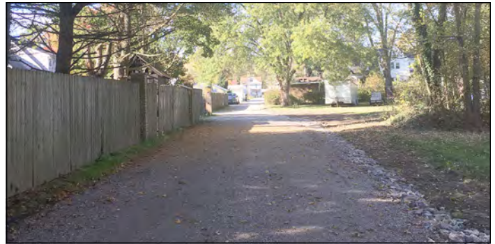
BERRY ALLEY READY FOR FUTURE PAVING
